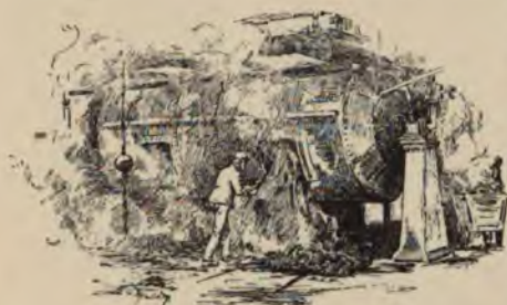
RAKING OUT A CYLINDER.
